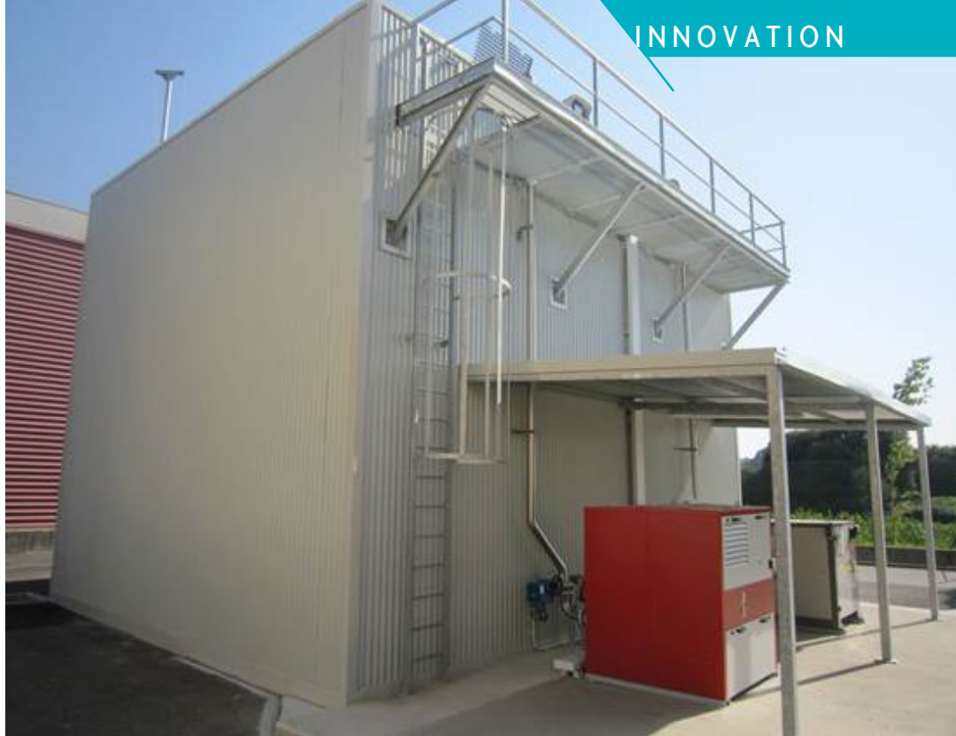
Exterior appearance of the building that houses the buried homogenization tank and the two ELAN® reactors of which the project consists.
